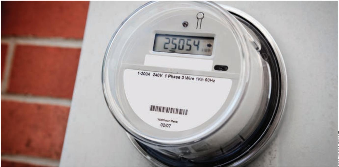
**FOR THE PAST 20 YEARS, TRI-COUNTY ELECTRIC COOPERATIVE** has operated on an automatic meter reading system with digital meters. This system requires meter reader personnel to travel to member-consumers' homes each month with portable data collectors to manually retrieve monthly kilowatt-hour usage.
