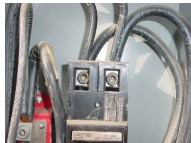
Double Tapped Wires
