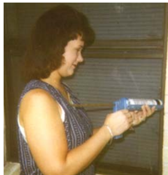
A little time spent with a caulk gun and scraper can save energy and prevent costly repairs from water damage. Take a look at your windows, doors and plumbing penetrations and make sure they are sealed.
